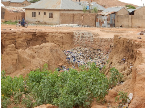
The culvert at Bagadaza
